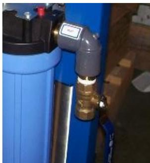
**Plumbing (*continued*):** Attach ½” hose to the ½” barbed fitting at the top back side of the product water flow meter using hose clamp.
